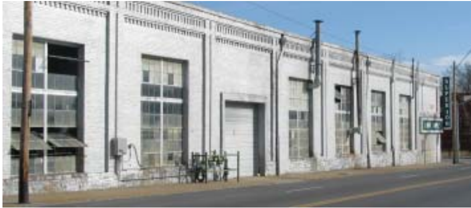
Another view of the plant, which once housed and provided power for electric trolley cars
