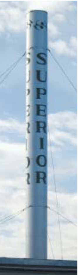
Unused stack builds brand ID.
