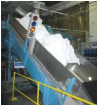
Soil goods move via conveyor into the tunnel washer.
